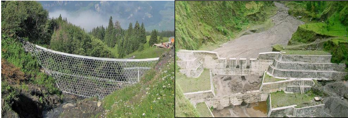
Gambar (Figure) 8. Contoh bangunan pengendali sedimen. Kiri tipe ringnet, kanan sabodam tipe terbuka (Sample of sediment control building. Left, ringnet barrier type. Right, open sabodam)
